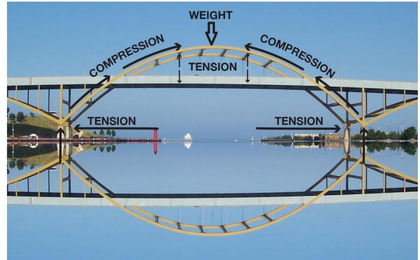
These investigations have focused on how triangles and arches can make a bridge stronger, but there are other shapes used in the bridges around our city. The Hoan Bridge and the Menomonee River Railroad Bridge look different, but the basic physics of them is the same. Each bridge uses shapes to do its job just right. Think about the different shapes and how they may be pulling or pushing on one another, each time you see a bridge in Milwaukee!
